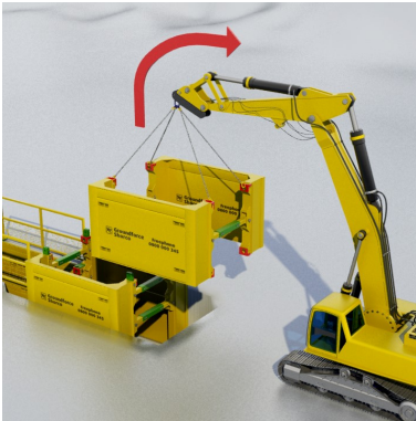
4. Attach a four leg lifting chain to the lifting points. Lift the top box clear and set carefully to one side.
