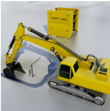
1. Excavate a nominal one metre deep guide trench.
