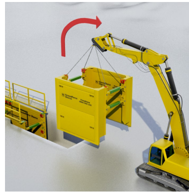
8. Attach a four leg chain to the lifting points and lift clear of the excavation.
