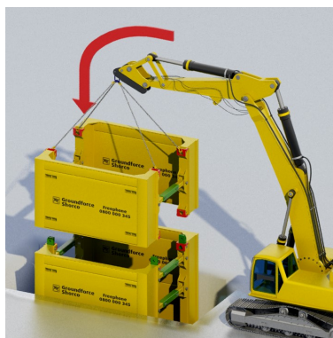
7. Prepare to fit the top box by raising it over the base box.
